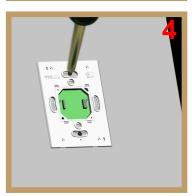
Remove the screws between back box and wall base
