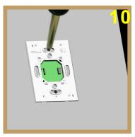
Tight the screws to the back box screw holes (can be installed in US back box, UK back box and Europe back box).
